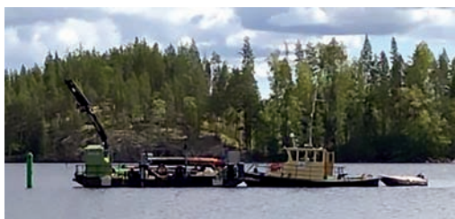
Installing smart buoys at the Finnish inland waterway. Source: Regional Council of North Karelia.
